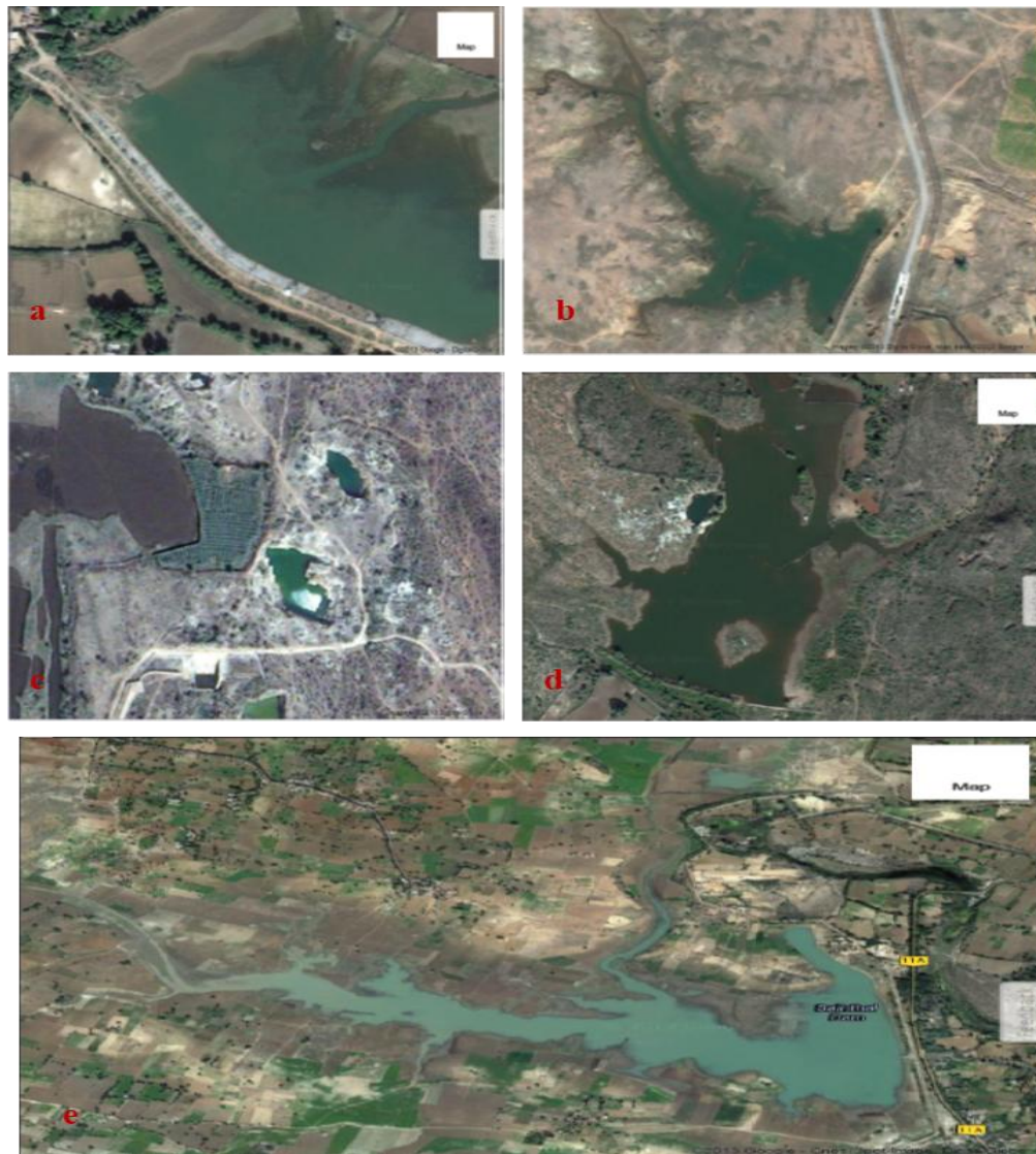
Figure.2 Google Earth images of various RWHS (a-d) and outlet of Arvari river catchment (e)
