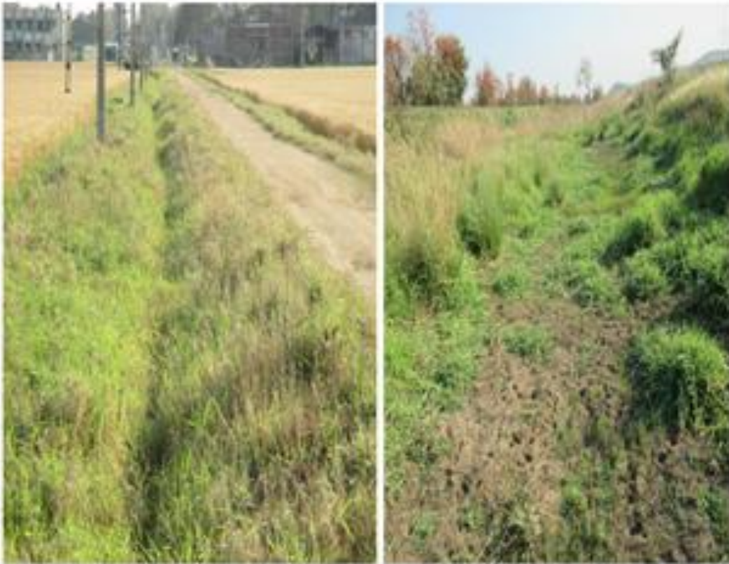
Figure.3 Drainage Line Condition of Area
