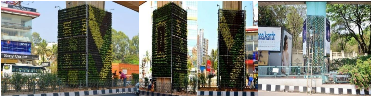
Fig.1 Installation of vertical gardens on metro pillars in Bengaluru for pollution control
