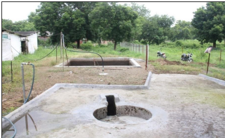
Fig.4 Installed 50 m 3 modified Janta fixed dome biogas plant
